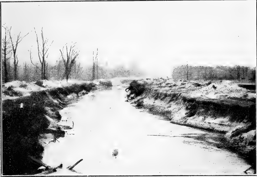
FIG. 1.—SLOPE COURSE OF SOUTH FORKED DEER RIVER DREDGED CHANNEL AT CAMPBELL'S LEVEE, NEAR JACKSON, TENN., 1916. (SEE TABLE NO. 3.)
